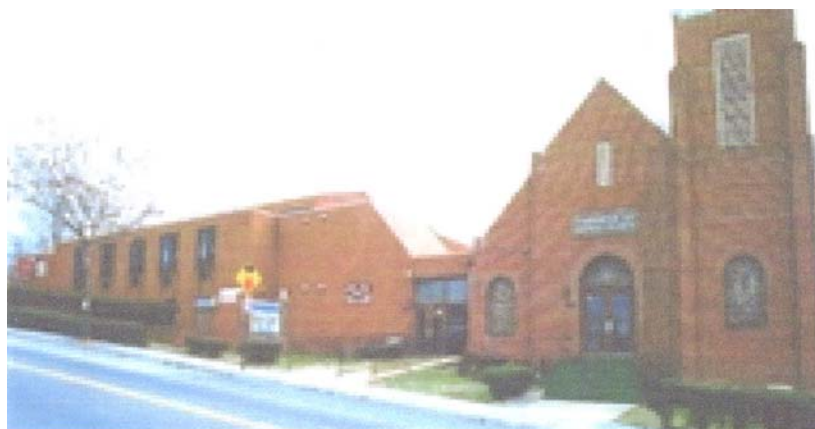
Our Present Church Building
